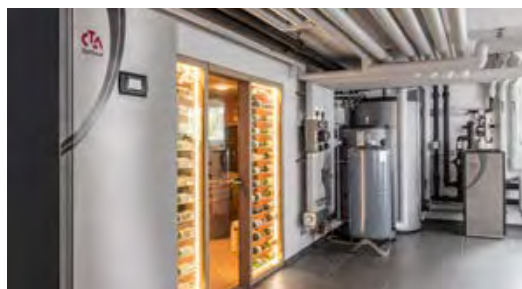
Connection to DHW storage tank, buffer tank and with „free cooling“. The heat pump is connected to geothermal probes.
